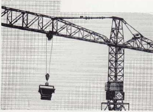
The filled skip is hoisted by the crane.
