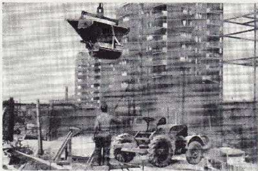
The empty skip is lowered on to a vacant Ground Frame.
